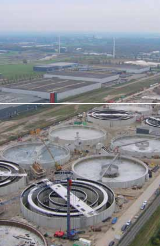
Wastewater treatment plant in Amsterdam - realisation with concrete protective liners.
