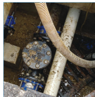
Pressure sewage main before installation
