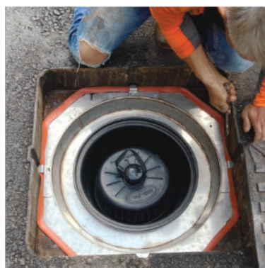
Installation is complete and a final seal check
