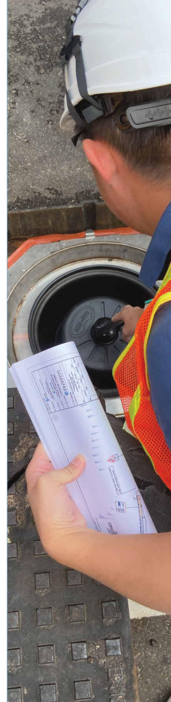
Pressure sewage main with the Odour Abatement Device frame installed
