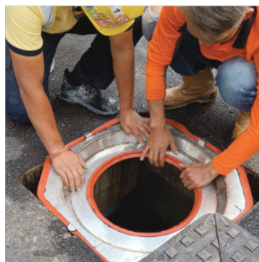
Placing the stainless steel frame
