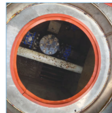
Pressure sewage main with the Odour Abatement Device frame installed
