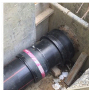
Pipe fused to transition, ready for encasement
