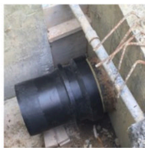
Installation of Transition c/w Puddle flange
