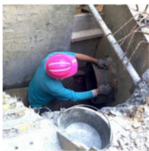
Preparation & measuring of DI Spigot
